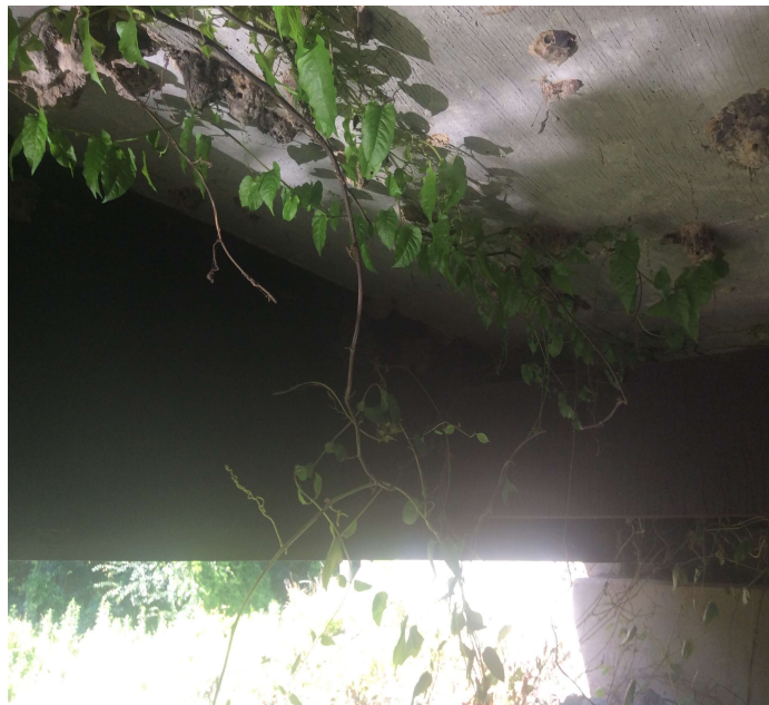
PHOTO 1 Description Span 1 vines growing on the underside of bridge.
